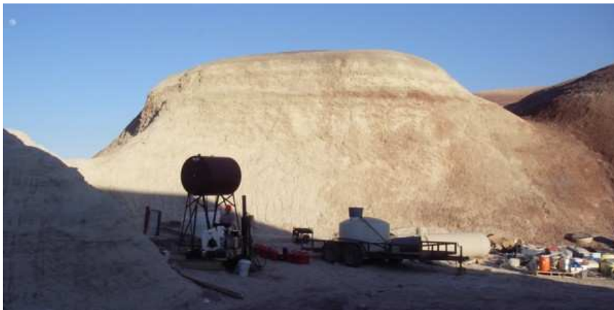
The engineering area from ground level with the power generator and its gasoline tank on the left. The ground water tank is located behind the tank tower. In the middle, the trailer with the water tank brought weekly from Hanksville.
