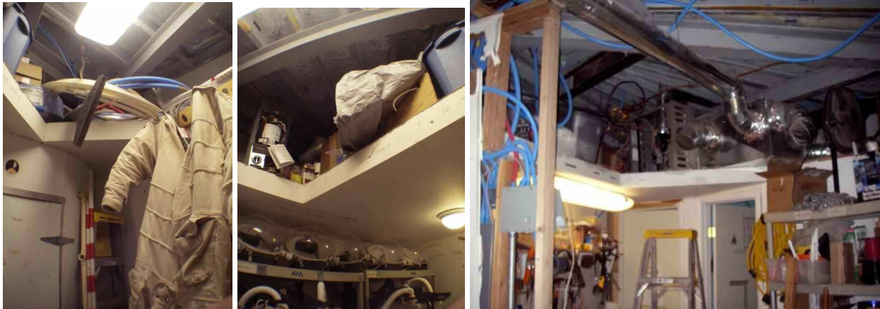
Storages areas above human height on the first floor. On the right the heating system.
