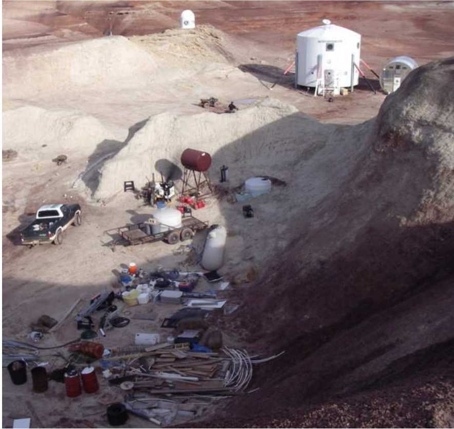
General view of the MDRS facilities. In the upper part from left to right: the astronomical observatory, the Hab with the main entrance to airlock n°1 and the greenhab. In the middle: the power generator with its gasoline brown tank on a tower, the ground water tank on the left, the water tank brought weekly to feed the previous one, and the horizontal grey propane tank for Hab heating. In front: the waste and unused hardware “Antartica” style.
